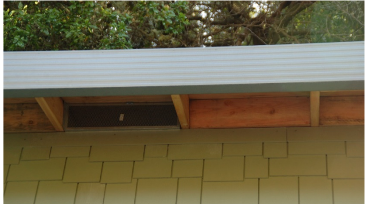
Figure 6.3. Vent located in the blocking space in open-eave construction. Photo: Stephen L. Quarles
