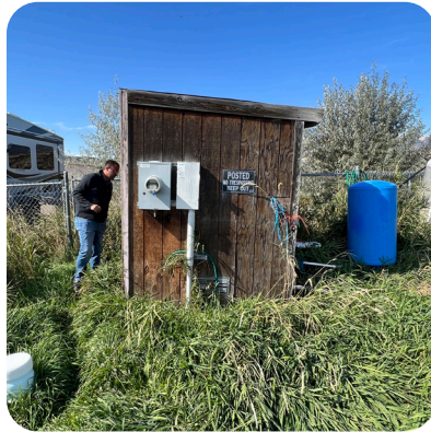
Irrigation Pump House
