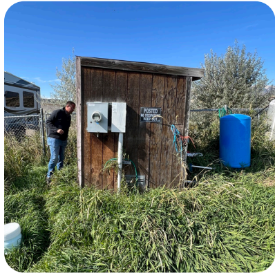
Irrigation Pump House
