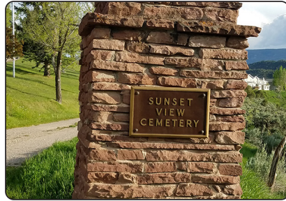
PLAQUE ON EXISTING PILLAR
