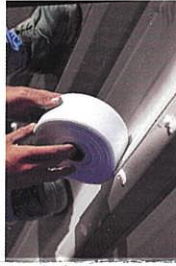
4. Reinforce existing seams with Spunflex® and base coat.
