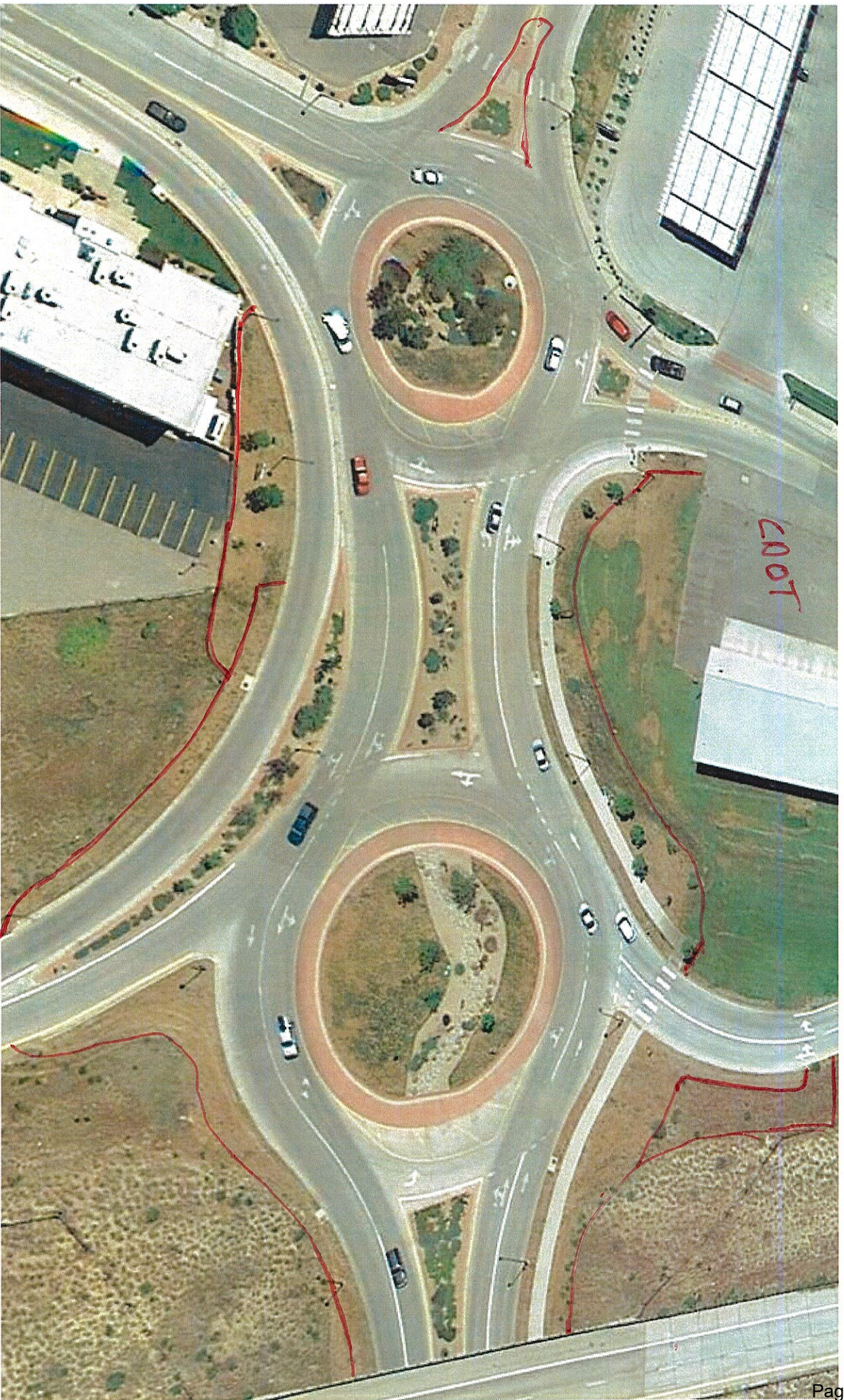
Roundabout area South of I-70
