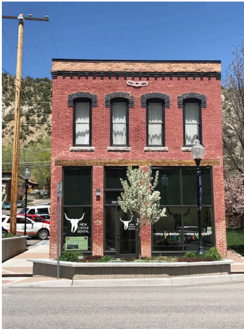
Odd Fellows Hall after renovation.
