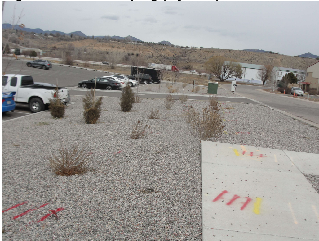
Along Enterprise Court
