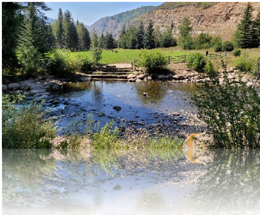
Designed step pool, access steps, and riparian restoration Vail, CO
