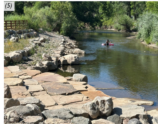
RiverRestoration River Access examples: (1) Boulder terracing (2) Soft access steps (3) Accessible wading ramp (4) Swimming hole (5) Hard access steps (6) Sandy beach
