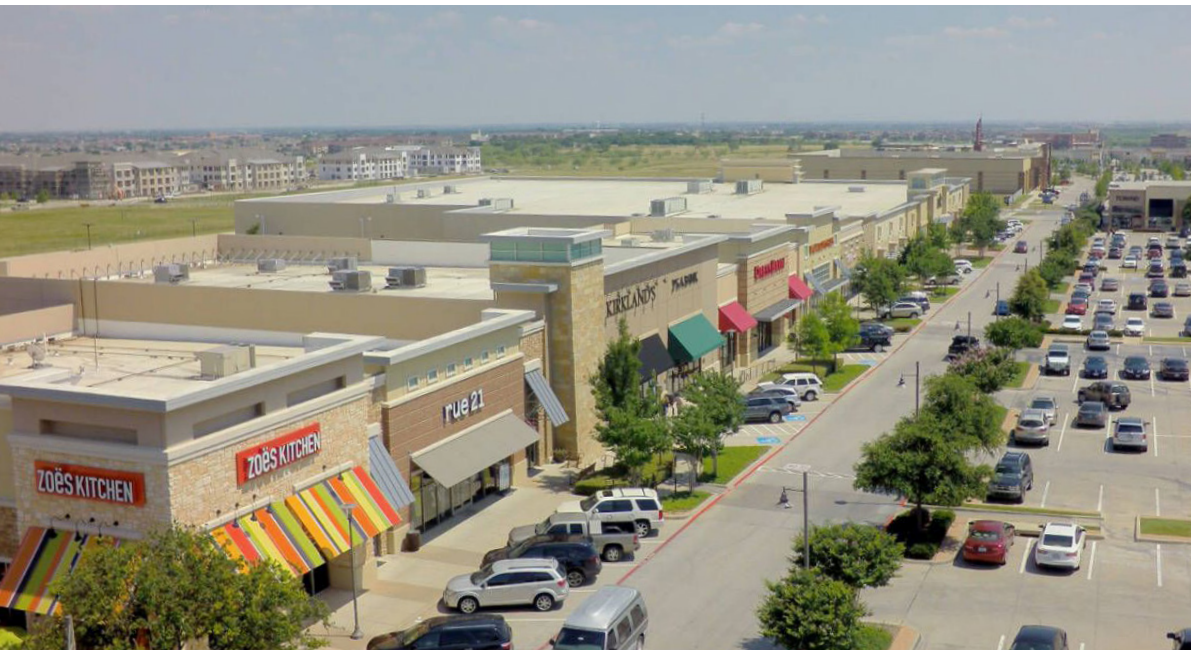
Retail area in AllianceTexas. (Credit: Heritage Homes )
