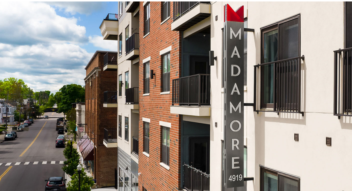
This mixed-use development, completed in 2020, is one of the largest investments Madisonville has seen in years. (Credit: Al. Neyer, LLC )
