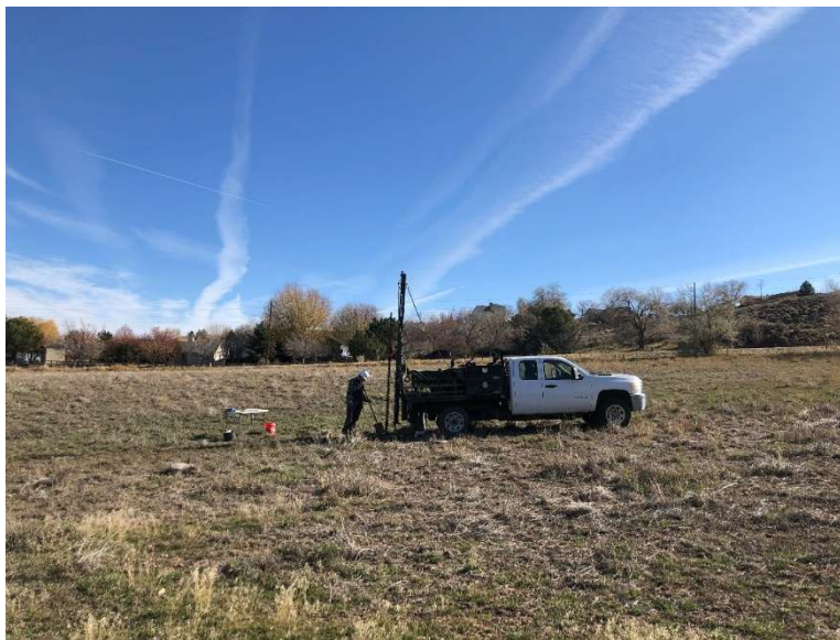
Figure 2 –Drilling Boring B-3, Looking East
