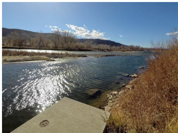
The Colorado River Near the Raw Water Intake Structure
