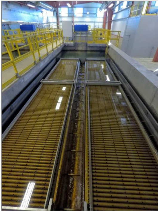
Plate Settlers in the West Sedimentation Basin
