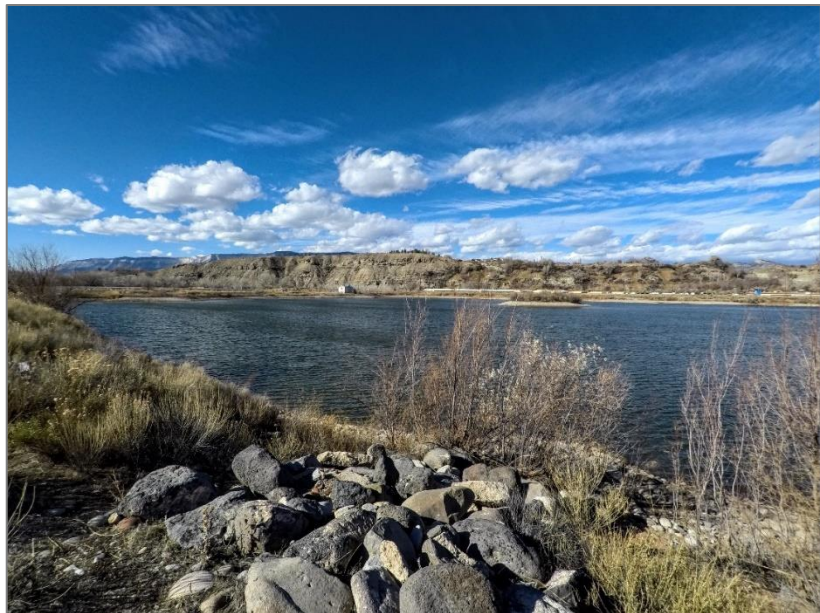
Raw Water Settling Pond with Raw Water Pump Station in the Background
