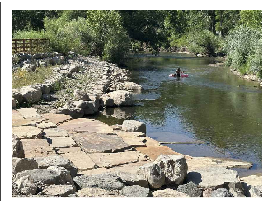
4a IMPROVED STREAM ACCESS – SLABSTONE TERRACE
