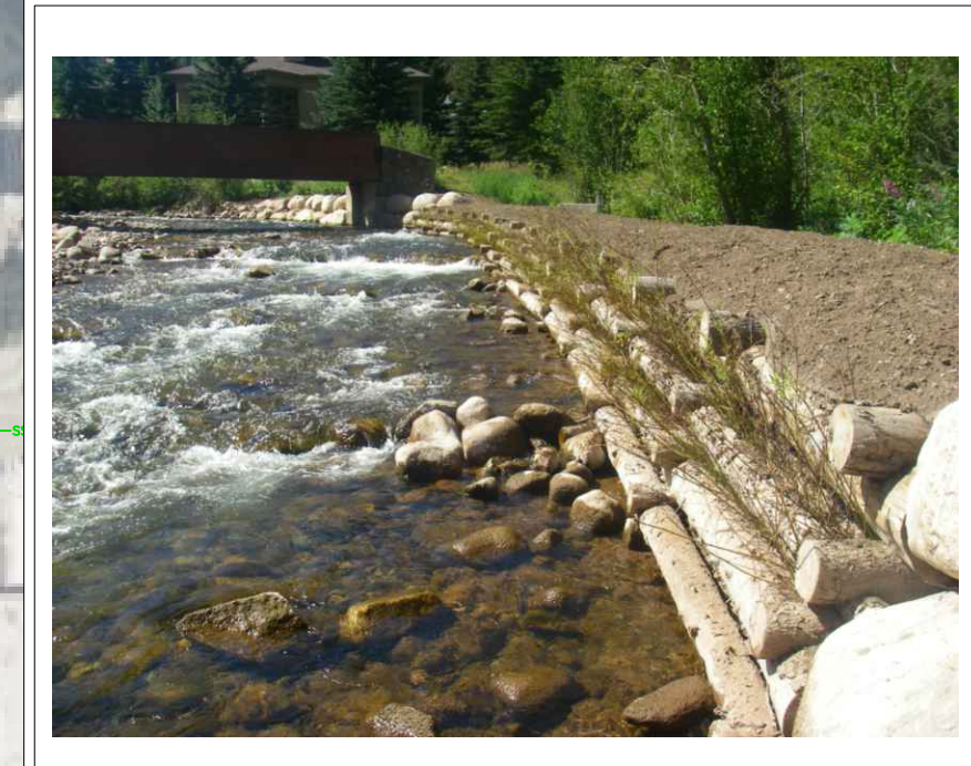
5 BANK STABILIZATION (BOULDER/LOGS)
