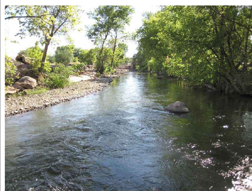
6 GENERAL CHANNEL GRADING & DEBRIS CLEANUP
