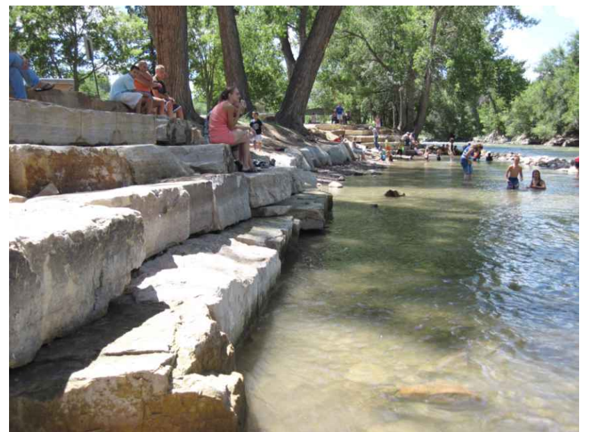
4d IMPROVED STREAM ACCESS – TERRACED BOULDER SEATING
