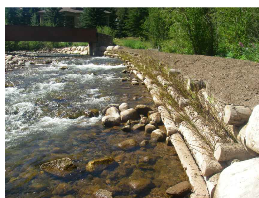
5 BANK STABILIZATION (BOULDER/LOGS)
