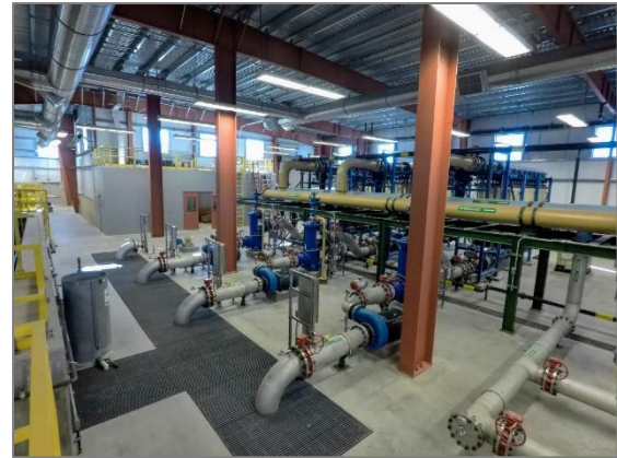
Pall Microza Membrane Filtration System
