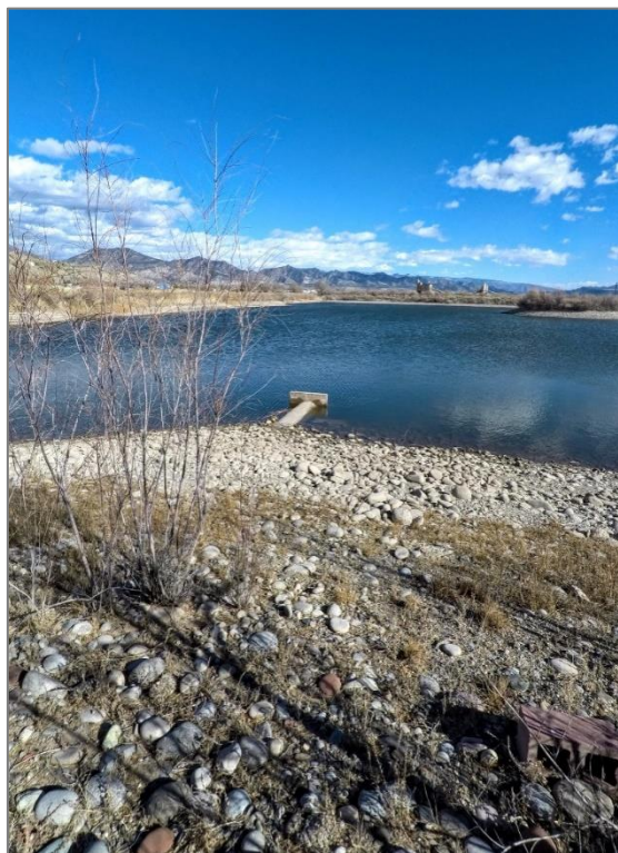
Raw Water Settling Pond Intake Pipe
