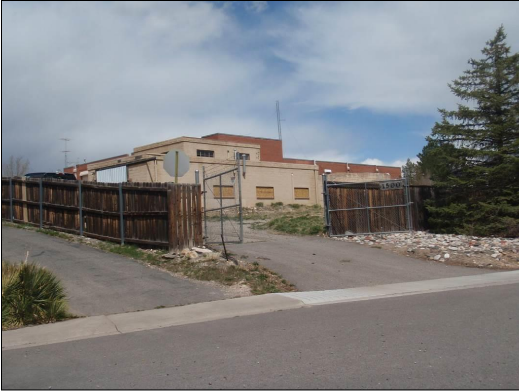
Former Water Plant Looking Northeast from Entrance at Dogwood Drive
