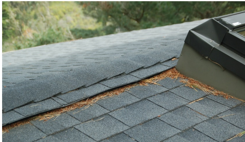
Figure 6.2. Debris accumulation at the entry of a (plastic) ridge vent. Ember ignition of this debris could result in ignition of the ridge vent. Photo: Stephen L. Quarles
