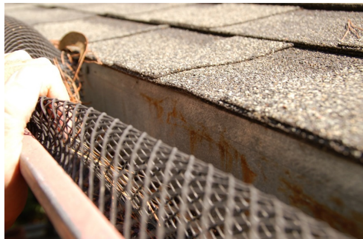
Figure 6.5 Metal drip edge installed at the edge of the roof. In this case, the drip edge was part of the gutter. Photo: Stephen L. Quarles
