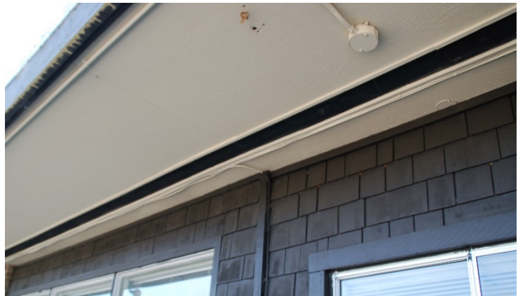
Figure 6.4. Under-eave strip vent located in a soffit. Photo: Stephen L. Quarles
